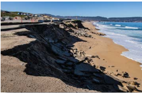
07-Coastal erosion of Del Monte Beach.JPG
