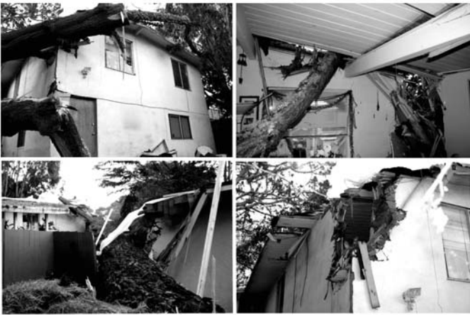
Fallen Tree Damages House during Storm
